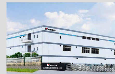
JIANGSU RAGOS PRODUCTION BASE
