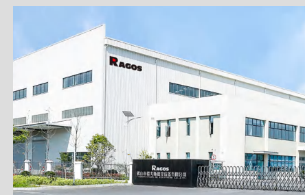
FOSHAN RAGOS PRODUCTION BASE
